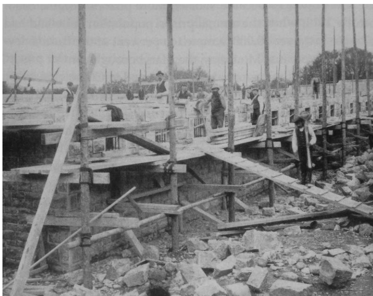
Figure 3.16: Construction of block E c.1899. 182
